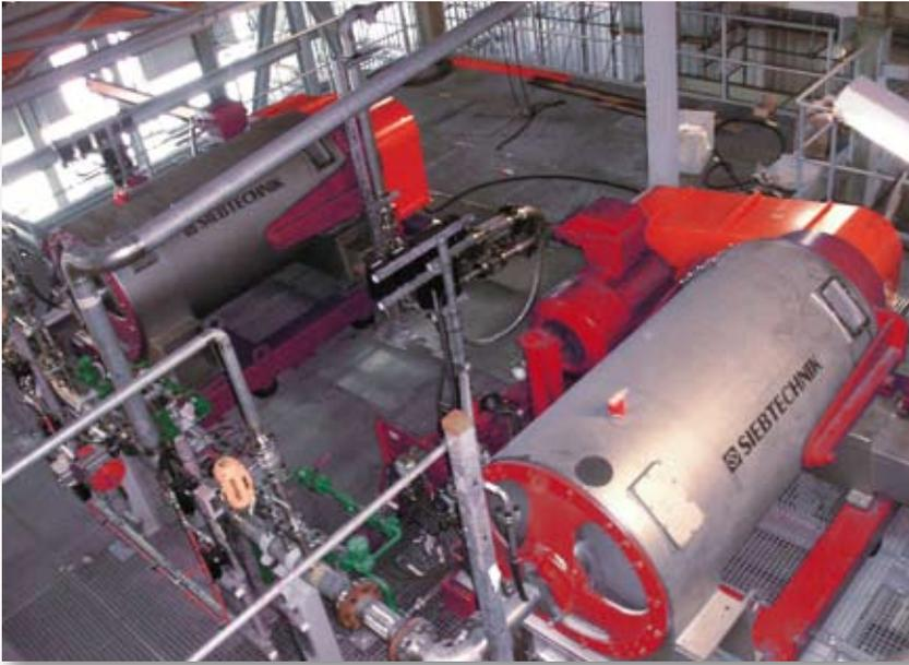
Decanters of the TS series are typically used in gastight process systems. The closed process housing in combination with proven sealing designs at the small shaft diameters and the design coordinated with the precise operating conditions give this centrifuge series a very high degree of reliability.
